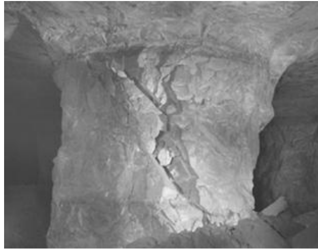
Figure 2-23 Instability of pillar between underground openings(Norwegian Tunnelling Society, 2016)
