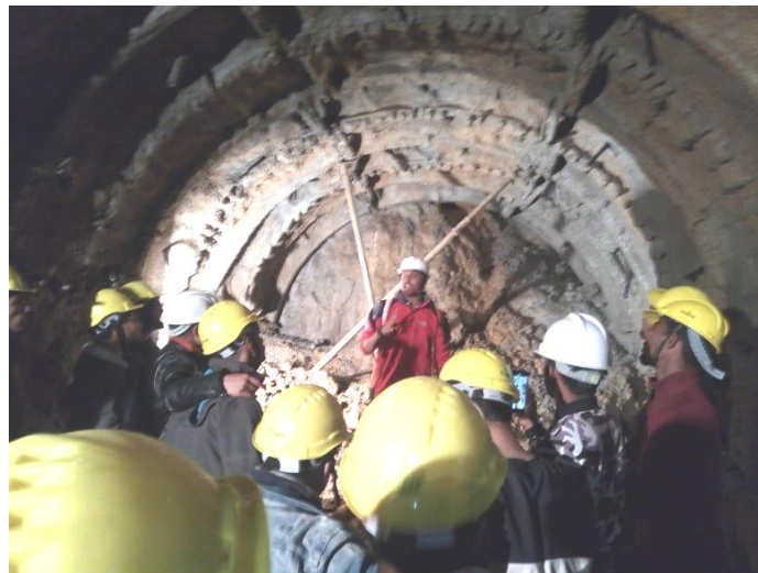
Figure 2-10 Use of Steel sets in weak, disintegrated rock at HRT of Super Madi
