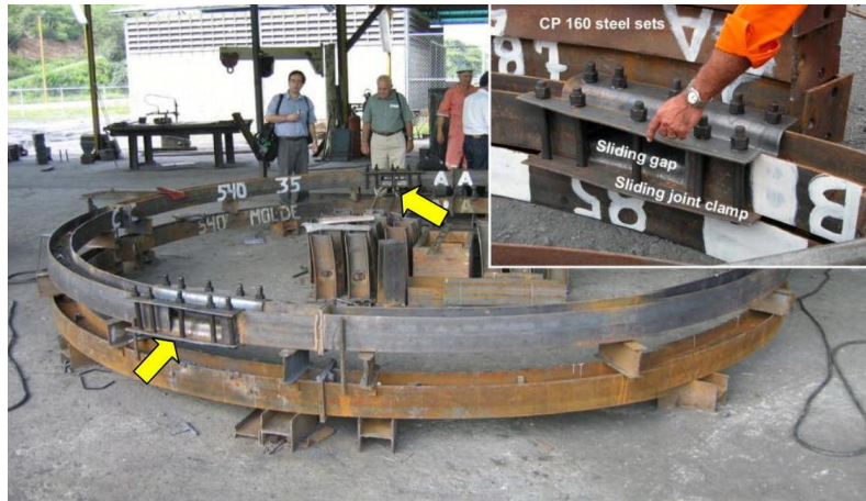
Figure 4-8 Yielding support with sliding gap present (Hoek, 2002)
