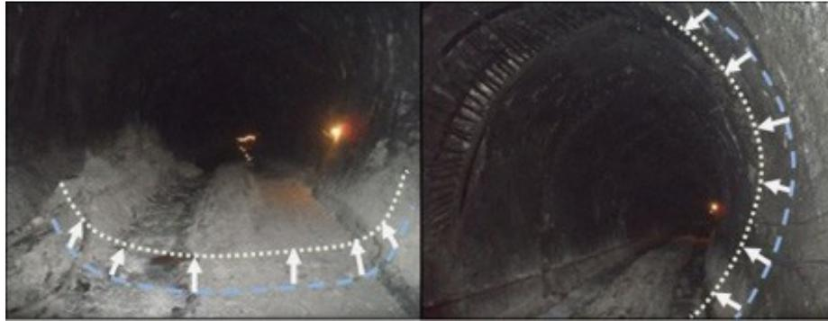
Figure 3-12 Tunnel squeezing Chameliya headrace tunnel. Floor heave (left) and wall closure in hill side (right) (Basnet et. al., 2013).
