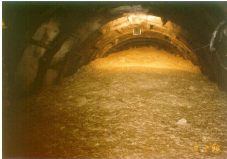
*Figure 3-6 Flowing mass from the tunnel crown (Himal Hydro, 2001)*
