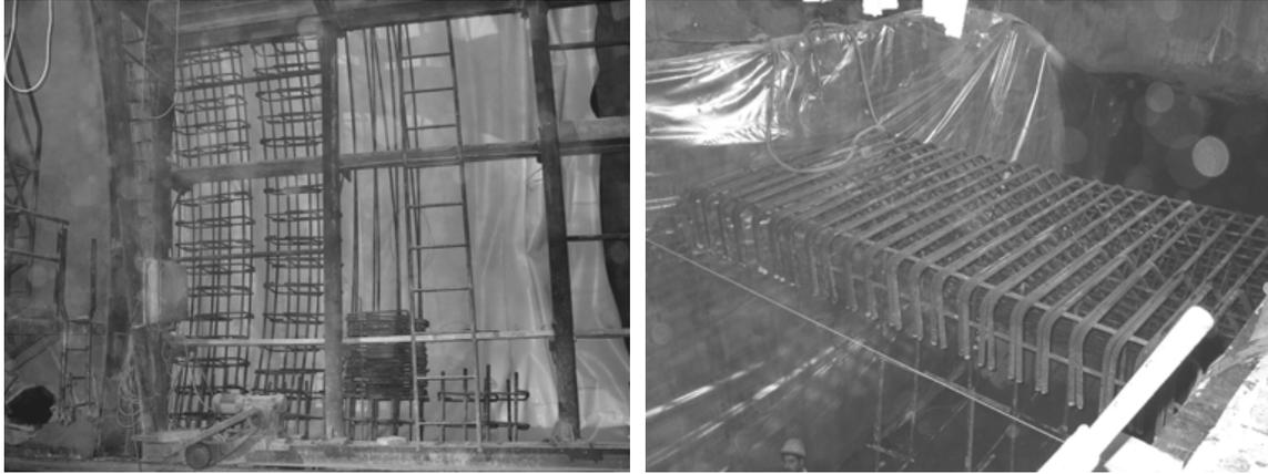
*Figure 2-16 Reinforcement details in lining at side wall and at invert (Russo et al.,2002)*
